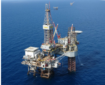
Figure 1 : Jackup Source: (Mudlogger (Admin.). 2008.)
